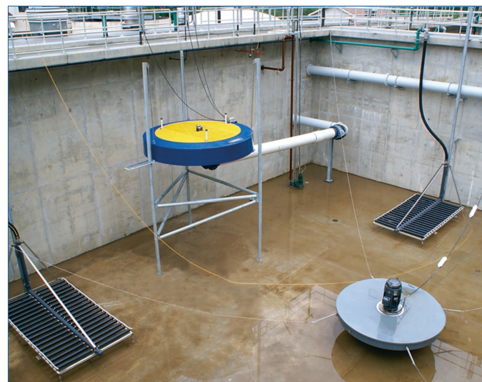
Full floor coverage diffused aeration is standard, optional retrievable diffusers are shown.
